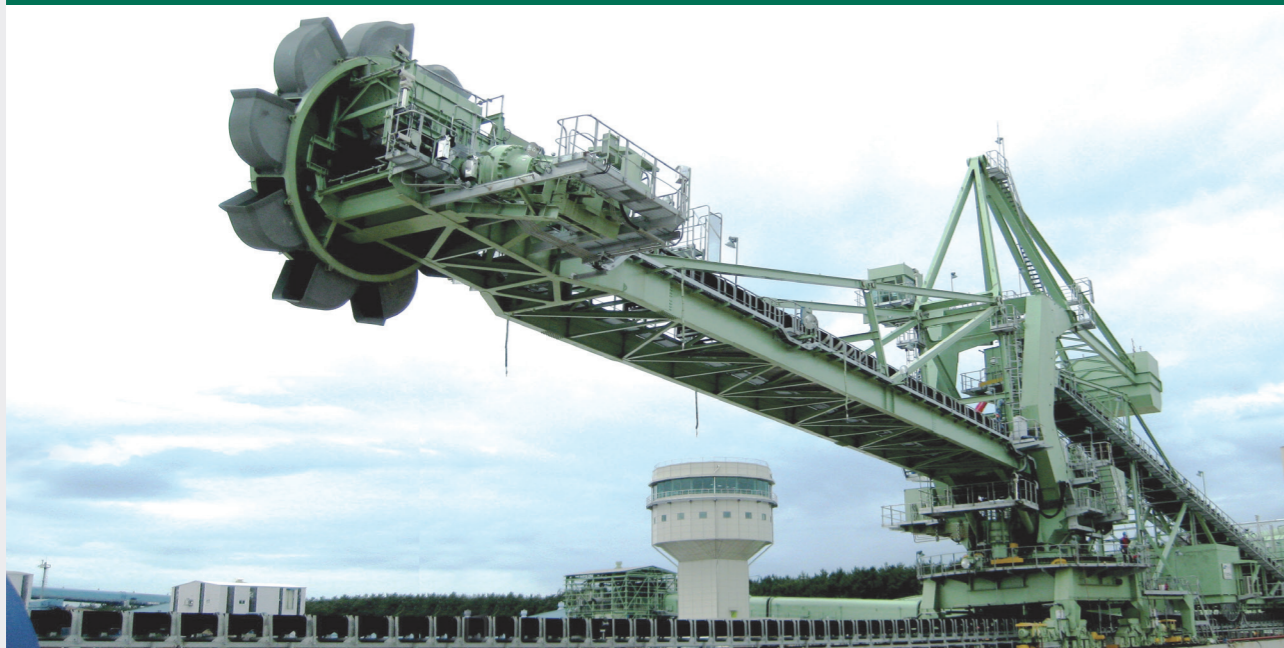
Yeongheung Thermal Power Plant : ST/RE 4800/4800t/h
