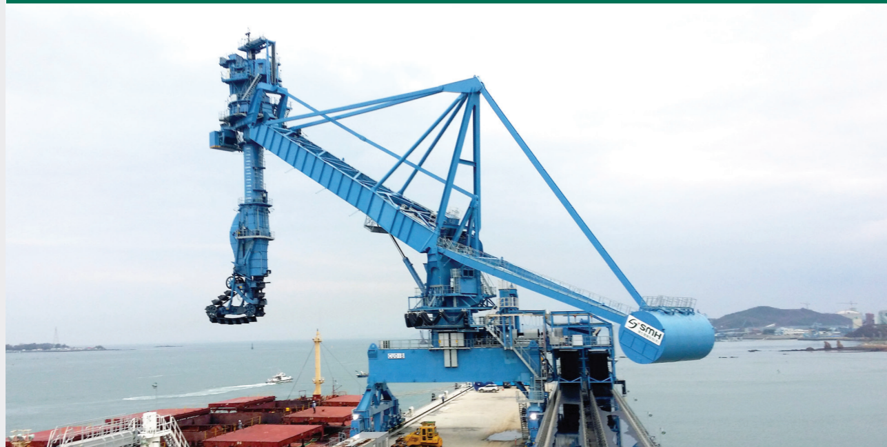
2700t/h CSU Sinboryeong NO.1,2 Coal Handling Facility
